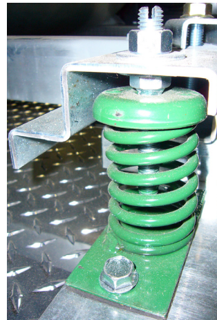
Figure 8: Spring Isolation
