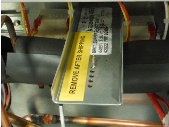
Figure 18: Compressor Brackets
