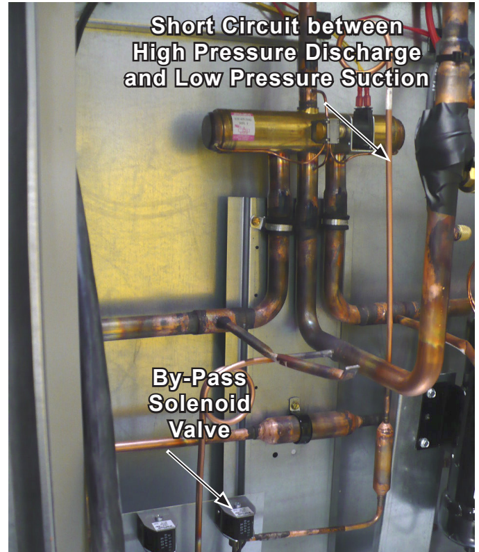
Figure 28: By-pass Solenoid Valve
