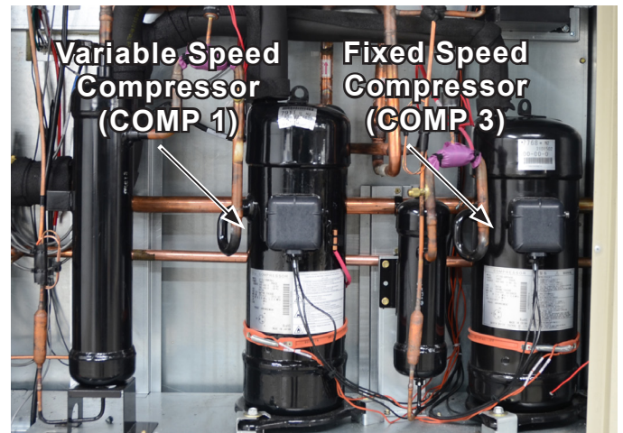
Figure 20: Compressor Tandem on Medium Cabinet
