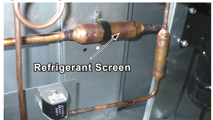
Figure 26: Refrigerant Screen
