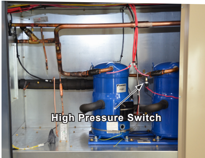
Figure 33: High Pressure Switch
