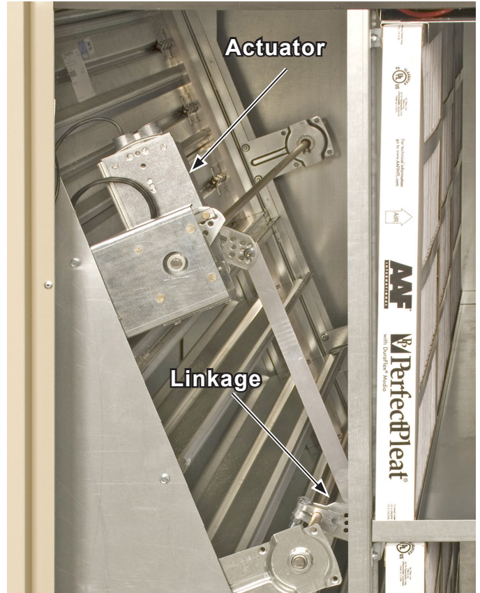
Figure 11: Damper Assembly
