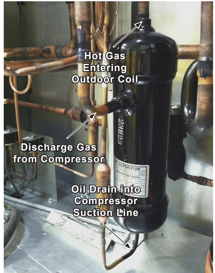
Figure 22: Oil Separator
