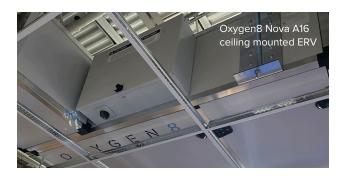
**New technology is available.** Using decentralized ventilation, each energy recovery unit delivers fresh, filtered outside air directly to the classroom, while stale air is exhausted. Decentralized ventilation eliminates the need for vertical duct chases, rooftop units and bulky equipment. Low-profile ERVs can be floor, wall or ceiling mounted to fit into drop ceilings and mechanical rooms with limited space.
